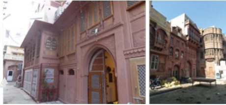
Figure 20 & 21: Conversion into hotel needed change as per requirement. A beautiful school building in use but need maintenance.
