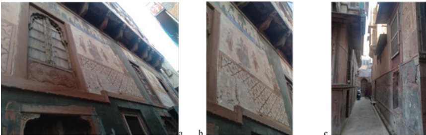
Figure 17a,b, & c: The frescoes of the walls were damaged due to pollution Source: Author
