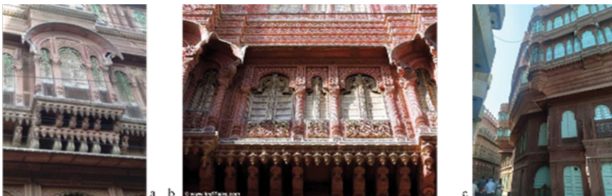
Figure 8a,b & c: Projected Jharokha with Chajwal & deep carving provides shade to the street
